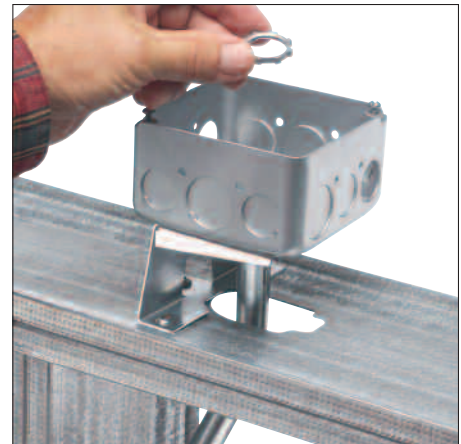
5 Install locknut on EMT fitting.
