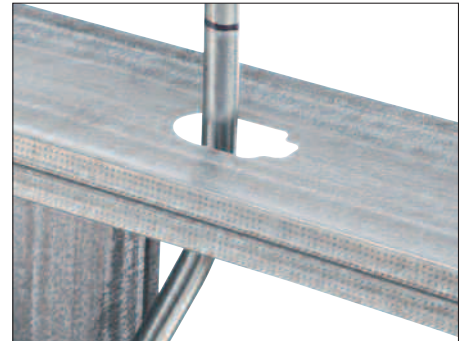
2 EMT marked and ready to cut.
