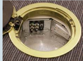
RFB6E configured for power and audio/video.
