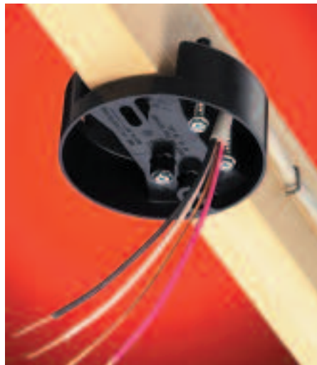
3 Pull NM cable through connector.
