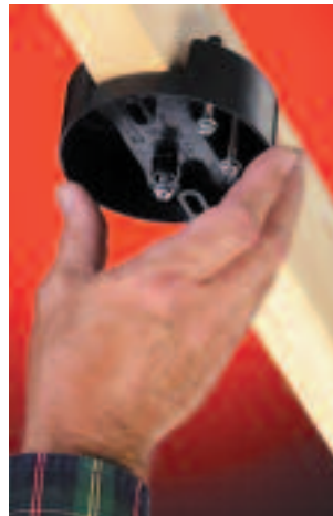
1 Press box onto joist.
