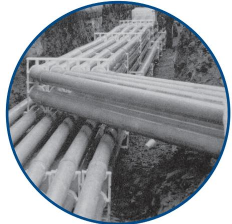
Nonmetallic Snap-Loc™ Spacers are designed specifically for use with nonmetallic duct, with maximum O.D. dimensions as specified in NEMA TC-2, TC-6 & 8, TC-10 and ASTM F512. The innovative vertical and horizontal interlocking Snap-Loc™ design has tapered joining slots with maximum tolerances for easy job site assembly.
